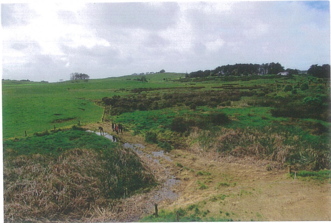
Photograph 3 Dam wall and stock access lane.
